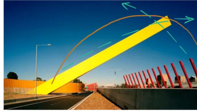
Melbourne International Gateway - arched and multiple component
