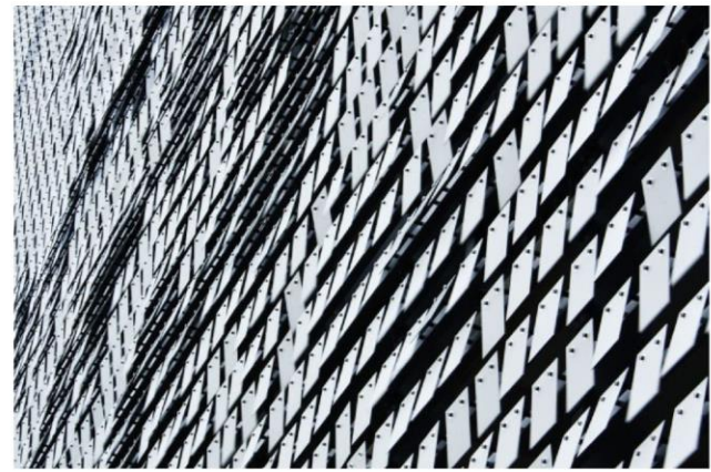
Turbulent Line , Artist: Ned Kahn, Brisbane Airport. A 5000 square meter kinetic façade, made by Urban Art Projects. Demonstrating how a simple mechanism can create gentle movement with the wind.
