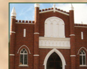
59 Mount Street Baptist Church Heritage listed (686) Federation Gothic
