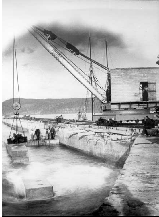
Figure 7 Constructing the Breakwater 47
