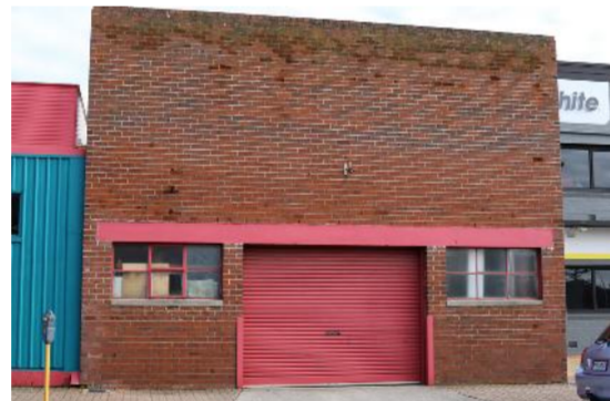
Warehouse along Mount Street
