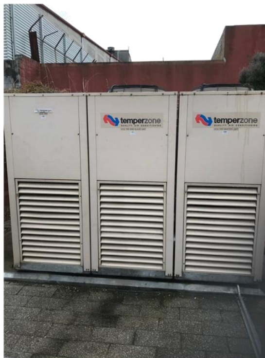
3 off existing modular reverse cycle chillers (Temperzone UCA 70R) to be replaced
