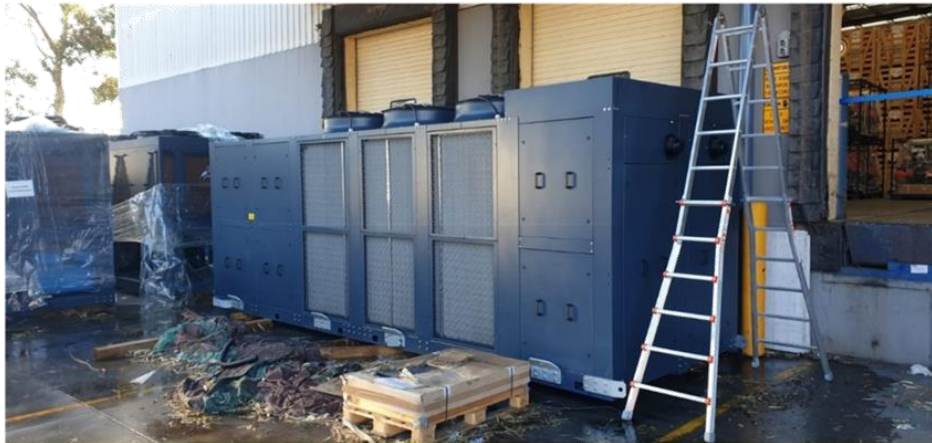
Proposed reverse cycle chiller unit (GeoClima VHA 2760 EC-01 HP TP) to be installed
