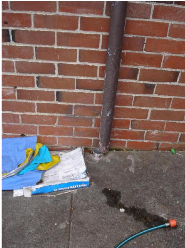
Photo 4. Misalignment of downpipe.
