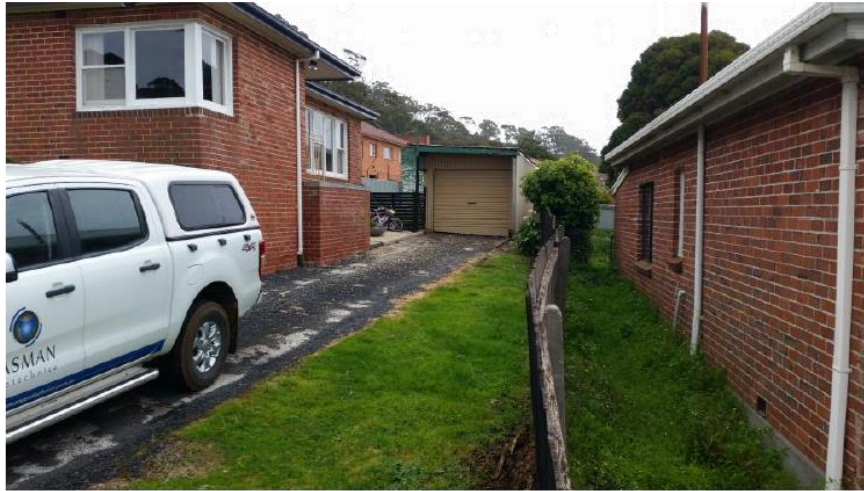
Photo 1. Leaning fence posts along the driveway.
