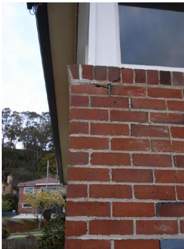
Photo 2. Cracks found on the existing dwelling.
