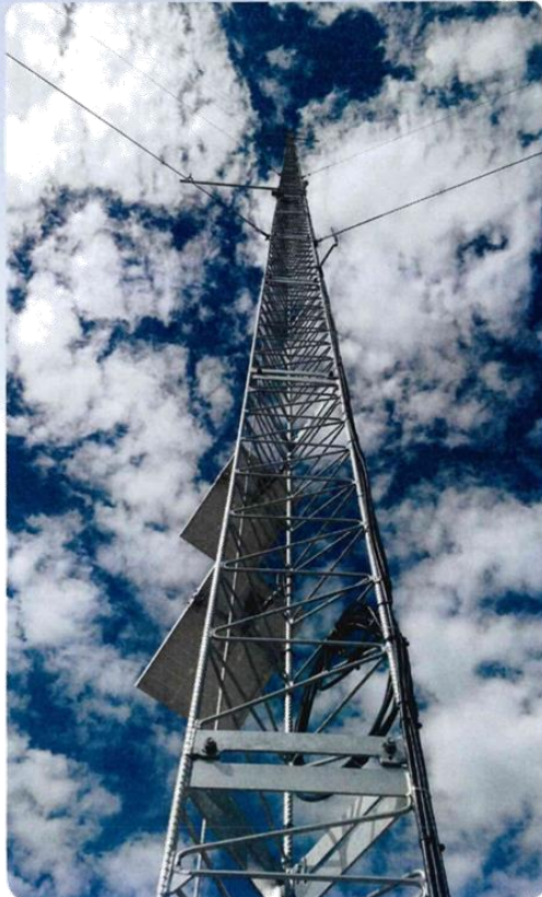
Installation is complete on the third meteorological mast on Robbins Island (photo credit: J Hammond)
