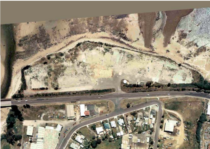
Figure 3e: c. 1996 shows demolition and new highway alignment BCC
